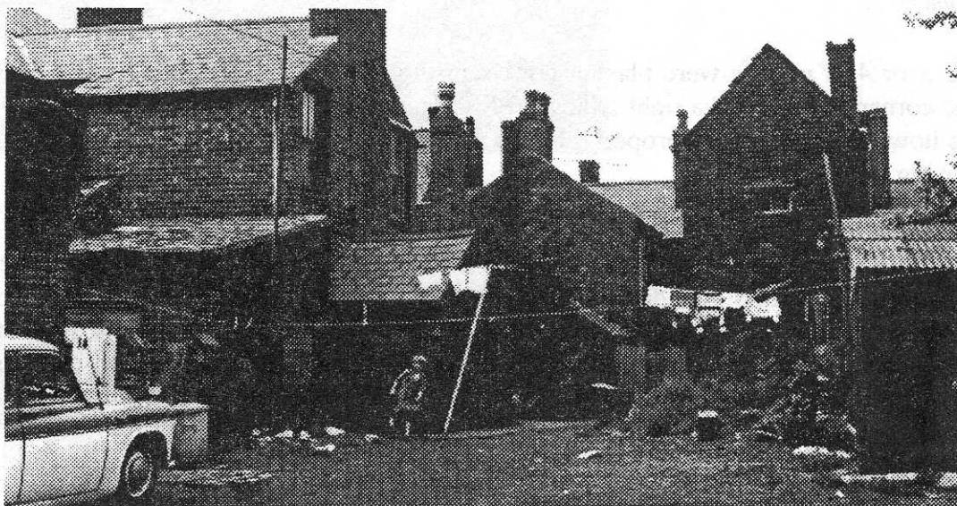
Langley Green - backs of houses before demolition in the re-development area 1970
